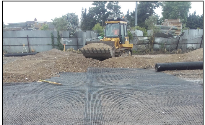
MacGrid EG40S laid with min 300mm roll overlap
