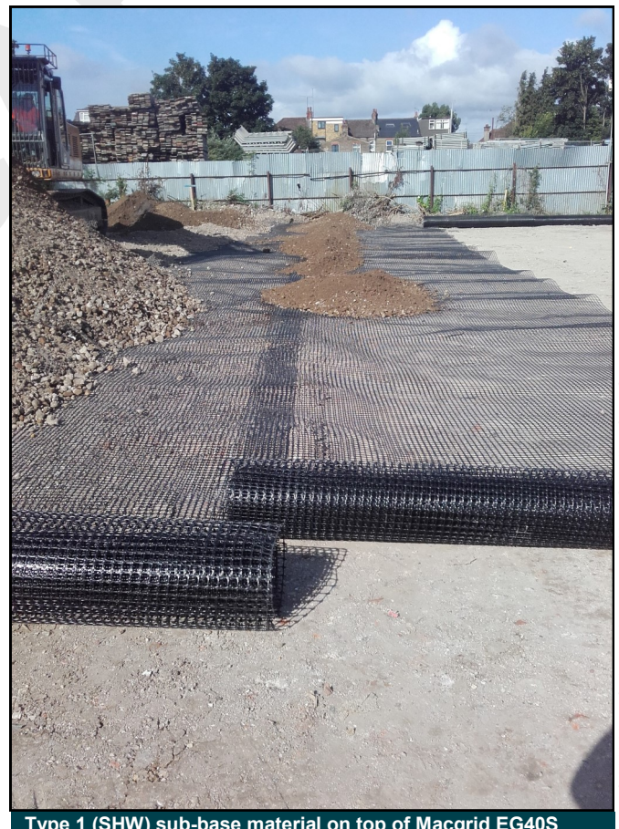
Type 1 (SHW) sub-base material on top of Macgrid EG40S
